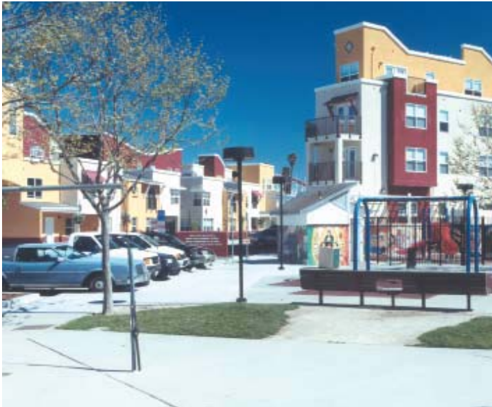
Located next to a city pocket park, the project includes a community center and child care center, paid for by the city, which also provided a 60-year land lease. Residents of the two- and three-bedroom apartments enjoy living environments filled with light, fresh air, and healthier interior finishes.
