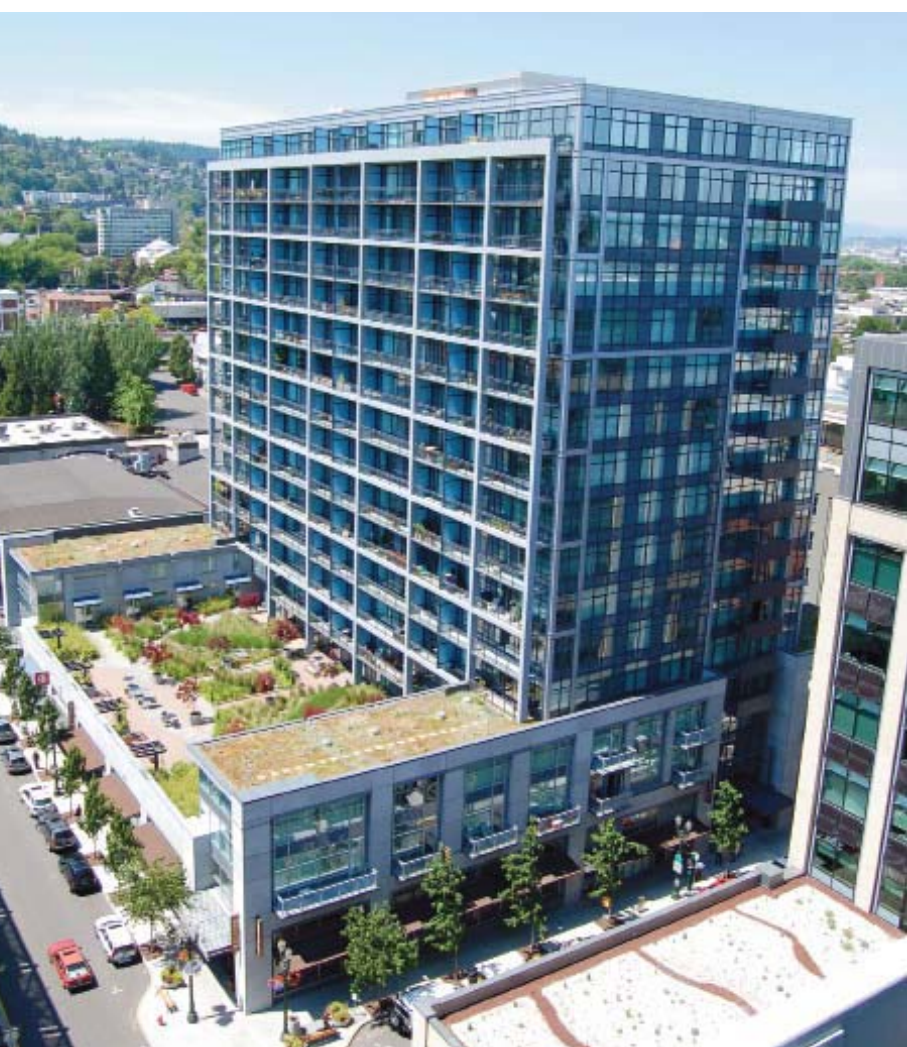
The Louisa Apartments in Portland, Oregon, completed in 2005, earned LEED Gold. Developer Gerding Edlen saved $40,000 in utility costs in the first year of operation.
