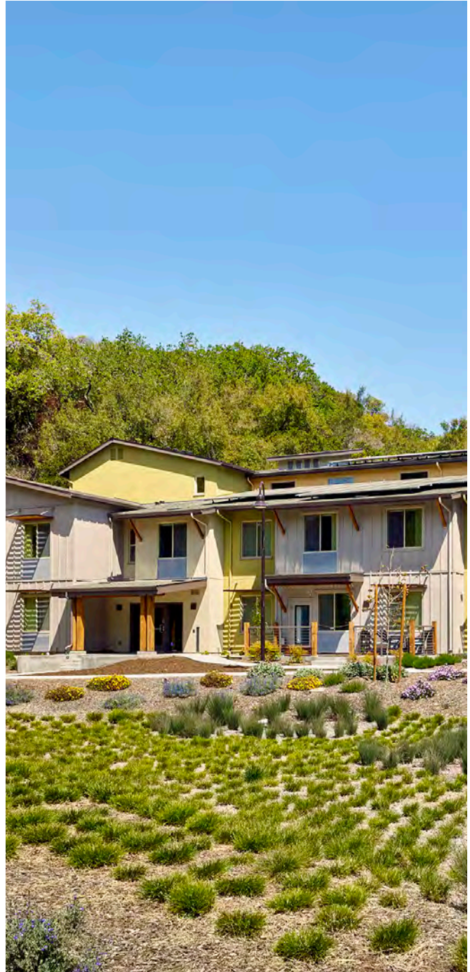
Our project in Marin County, a low income and formerly homeless senior housing development that was hard fought over for almost a decade, continued construction through the beginning of the pandemic, maintaining safety of the workers. Successfully completed, it welcomed its first residents in July of 2020 and served as a vaccination site for all the residents in the spring of 2021.
