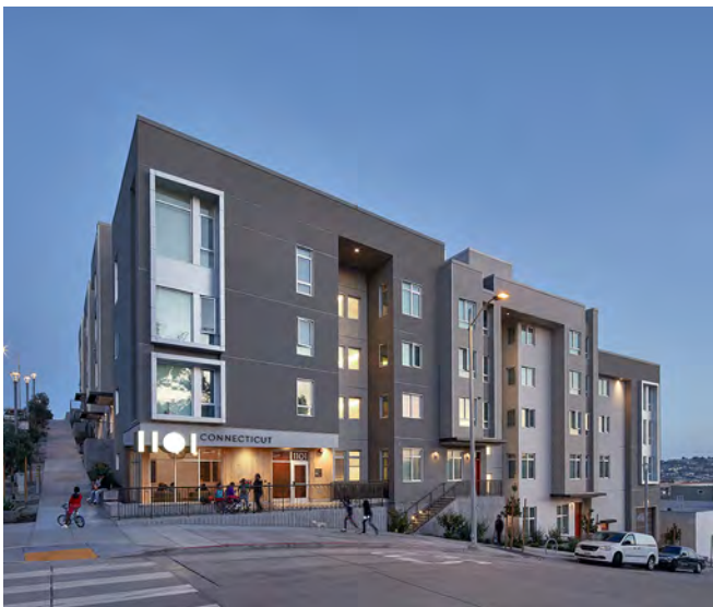
1101 Connecticut, San Francisco, CA: LEED Platinum - rooftop PV, solar thermal, 22k gal stormwater cistern, and 100% of stormwater treatment onsite.
