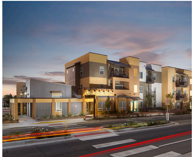
Del Corazón, Denver, CO: Enterprise Green Community - extensive use of photovoltaic panels, white TPO roof, air barrier building envelope, adjacent to public transportation, cement board siding, efficient windows and appliances.
