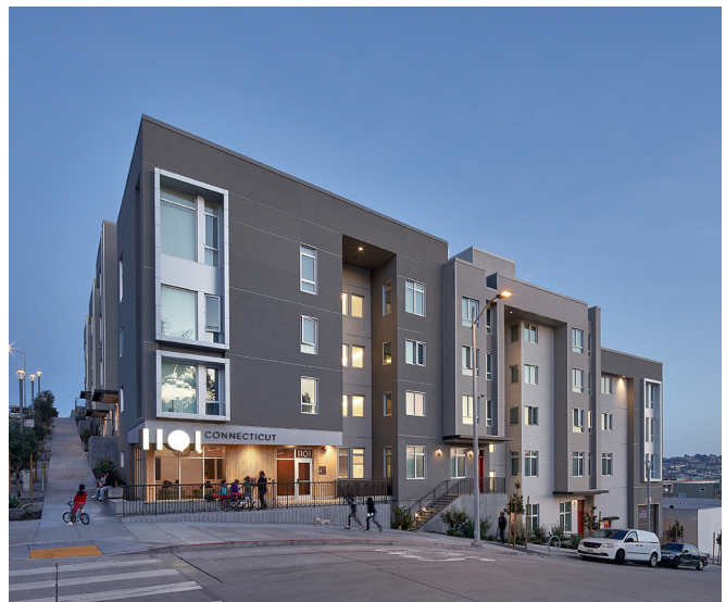
1101 Connecticut, San Francisco, CA: LEED Platinum - rooftop PV, solar thermal, 22k gal stormwater cistern, and 100% of stormwater treatment onsite.
